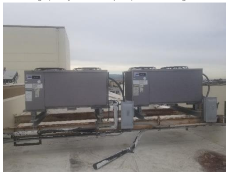
Existing split system heat pump outdoor units serving auditorium.
