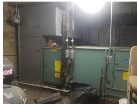
Existing split system heat pump AHU serving auditorium.
