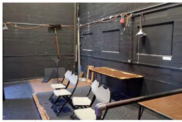
Plywood platform that raises tripping hazards
