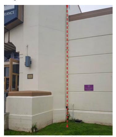
Seismic Separation at the Community Theatre (Seismic joint in red)
