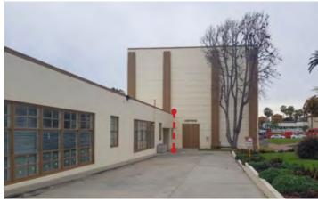
Seismic Separation at the Community Theatre (Seismic joint in red)
