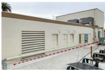
Seismic Separation at the Community Theatre (Seismic joint in red)
