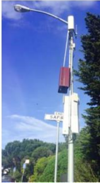
Exposed slack on cables and bulky equipment
