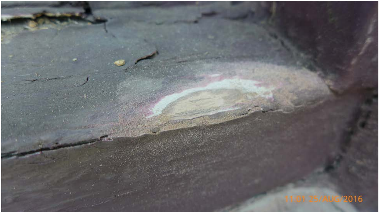
Window frame on west elevation of
