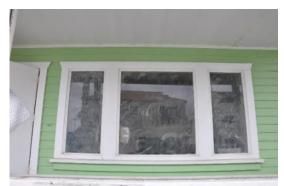
Figure 6: Tripartite window on each side of the main door with typical wood window surrounds that flare at the top.
