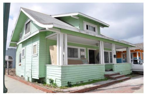
Figure 5. Front (north) façade of 70 10<sup>th</sup> Street with the flared eave and decorative ends to exposed roof beams. View looking southwest.
