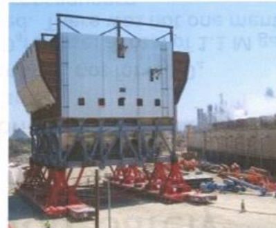
ESP being moved in 2008 to its final location
