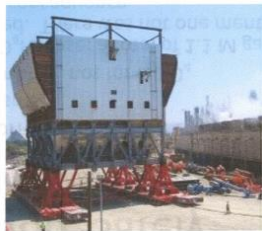
ESP being moved in 2008 to its final location
