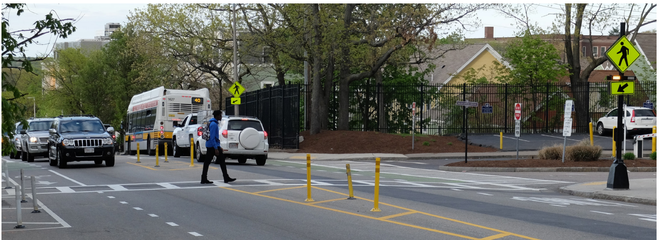
Under an on-call contract, we engineered the quick build of pedestrian crossing with Rectangular Rapid Flashing Beacons (RRFB).
