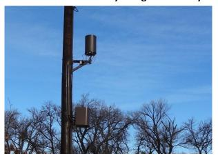
Cables are flush mounted and all equipment is painted to match pole
