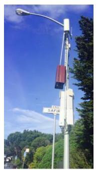
Exposed slack on cables and bulky equipment
