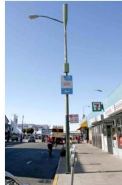
Lineal designed equipment and flush mounted on pole with colors to match pole
