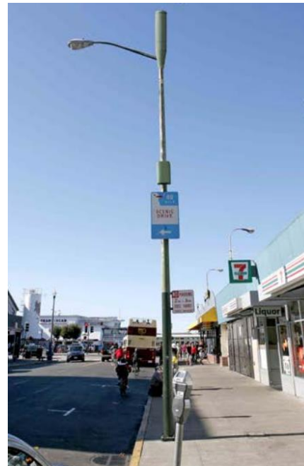
Lineal designed equipment and flush mounted on pole with colors to match pole
