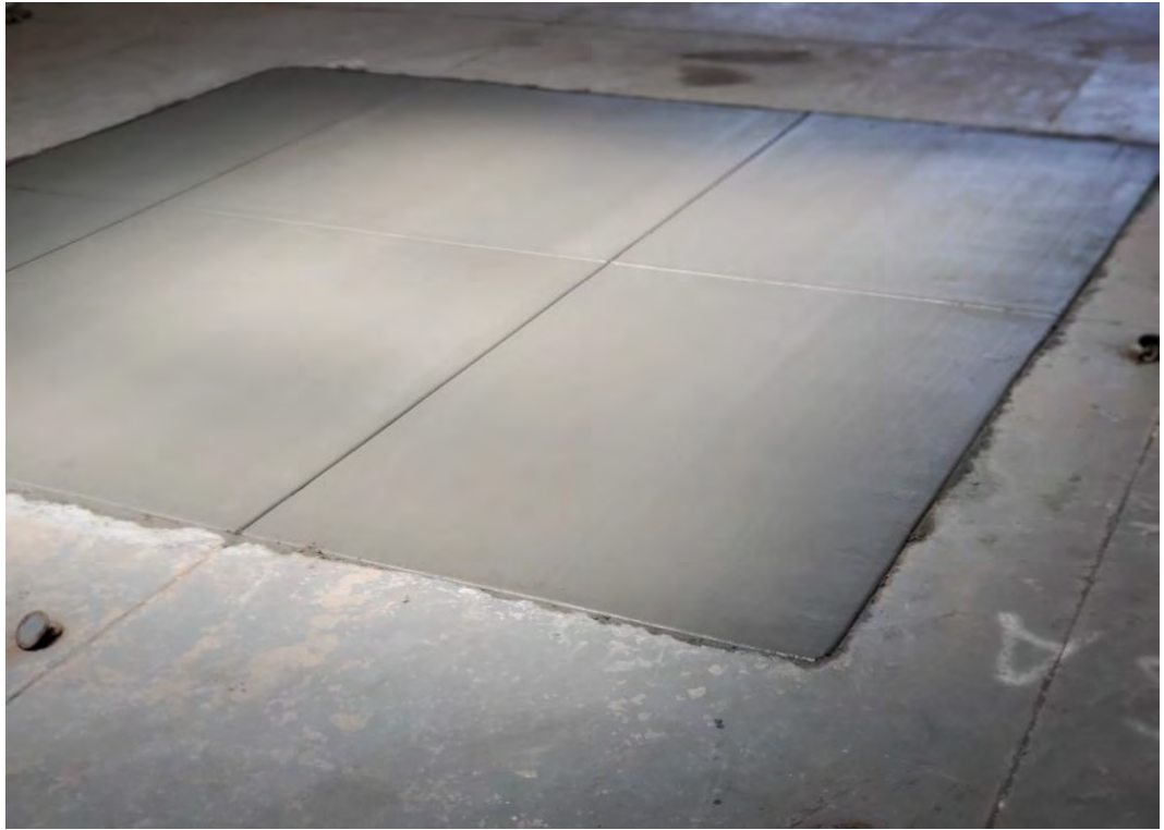
Concrete patch completed at Pit 1.
