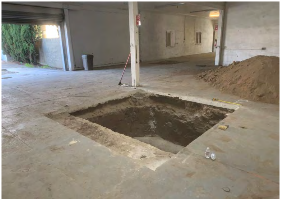
Pit 1 located in southwest corner of former shop building. No underground tank was observed in this location.
