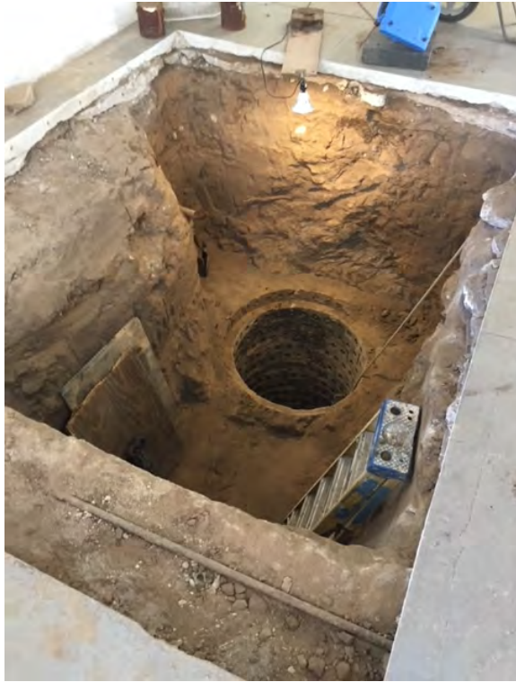
Pit 2 excavation and drywell location fully exposed and excavated.
