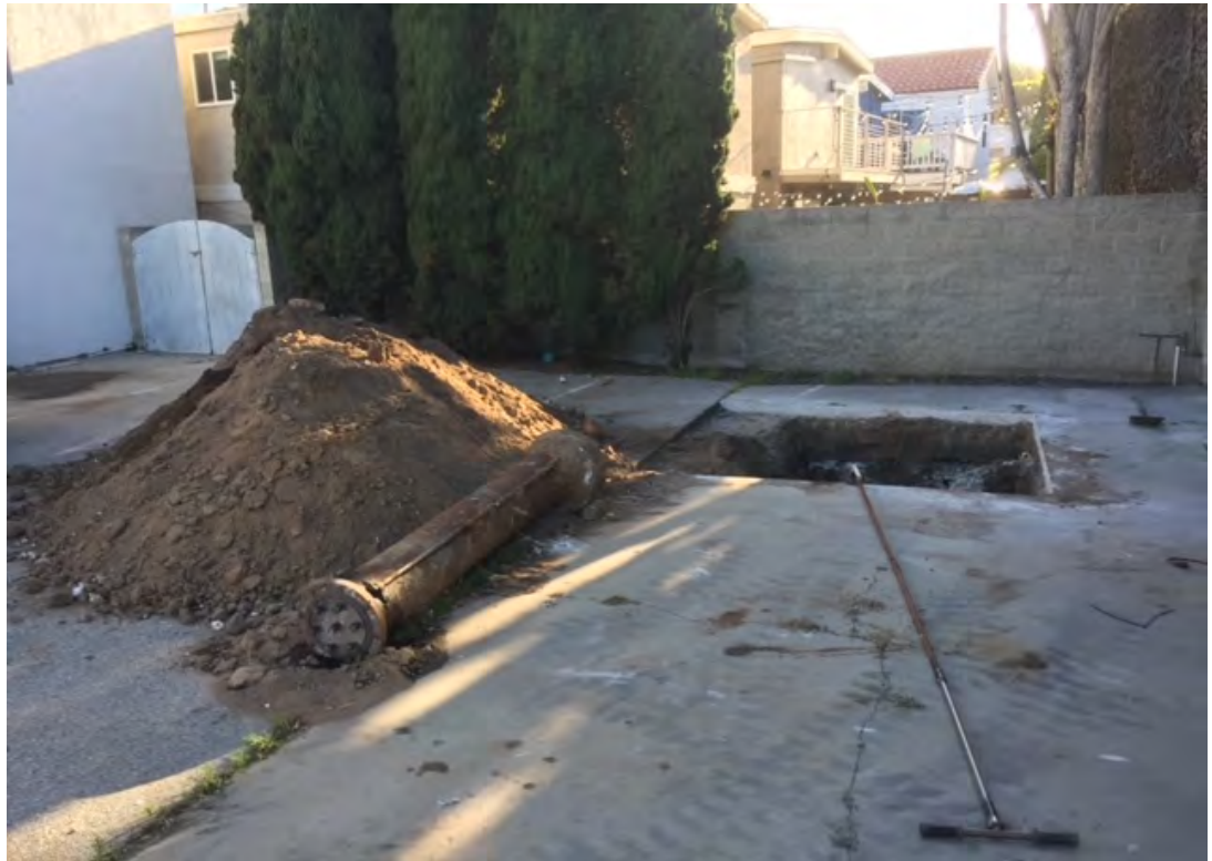
Hydraulic lift removal and excavation north of former shop building.
