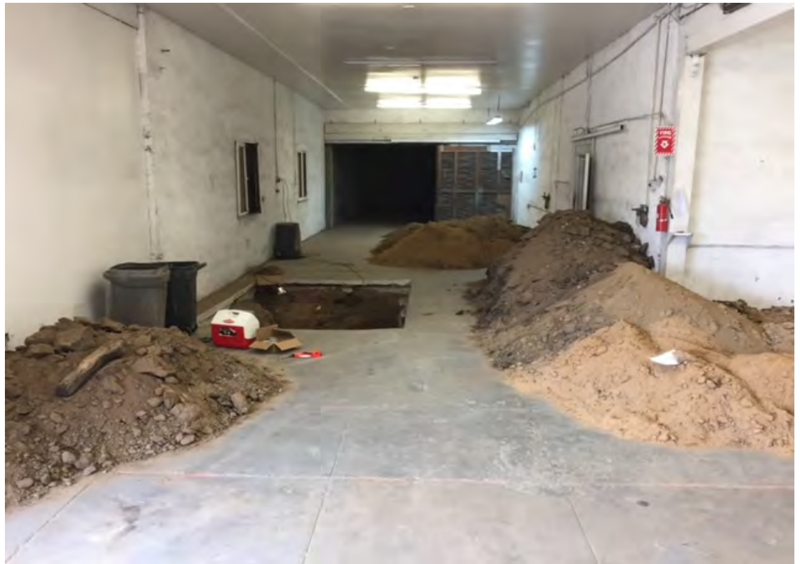
Soil stockpiles excavated from Pits 1 and 2 awaiting profiling for off-site disposal.
