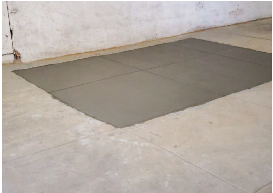
Concrete patch completed at Pit 2.
