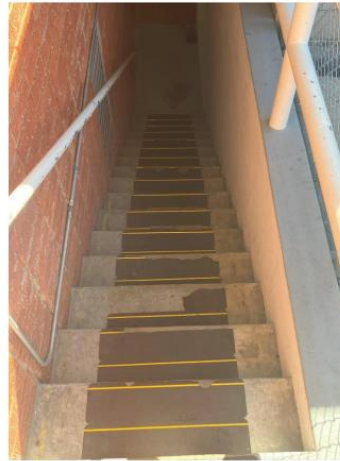
Gutters leak onto stairway
