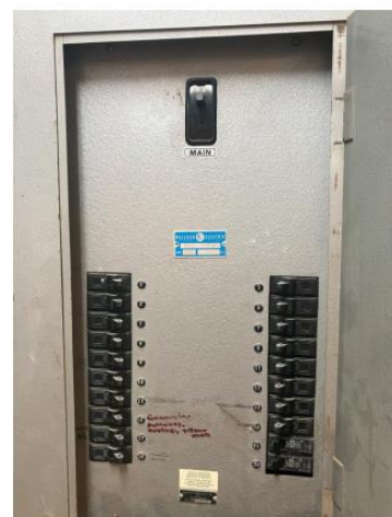
Electrical panels need to be upgraded
