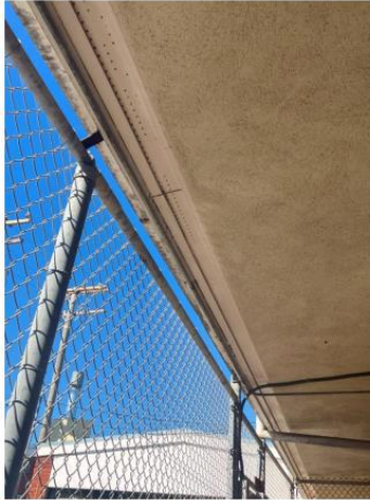
Gutters leak onto stairway
