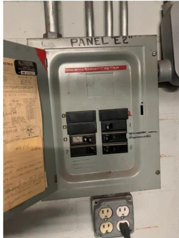
Electrical panels need to be upgraded
