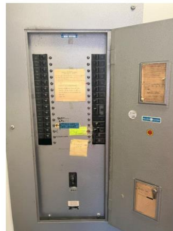
Old electrical panel needs to be upgraded
