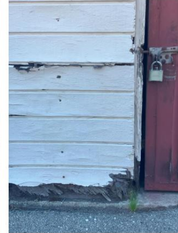
Water damage and wood rot
