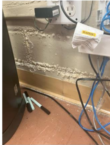
Mold on northeast wall (interior)
