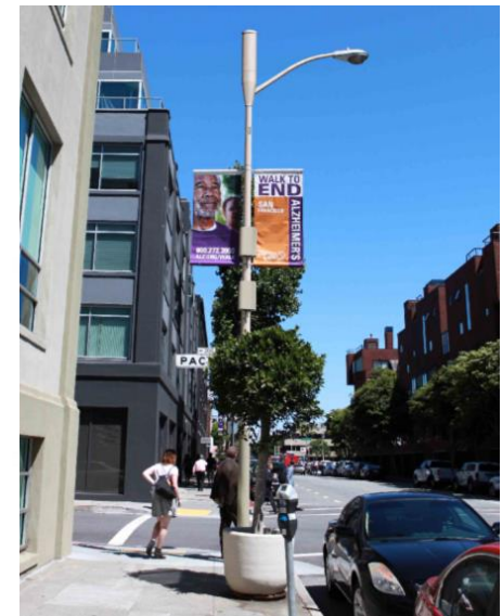
Lineal designed equipment and flush mounted on pole with colors to match pole
