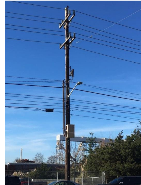
Cables and equipment are flush mounted and painted to match pole
