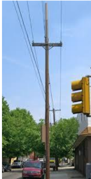
Cables and equipment are flush mounted and painted to match pole
