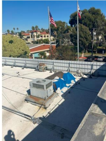
A/C Units and roofing
