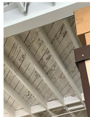
Roof leaking
